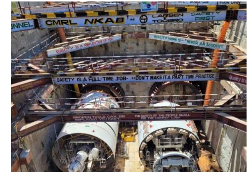
The finished waler brackets
