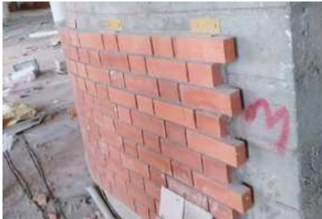
Application Details: Brick support connection
