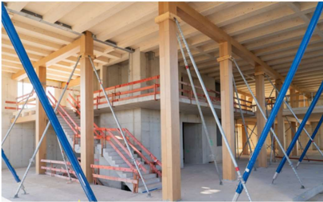
Application Details: Timber column connected to concrete
