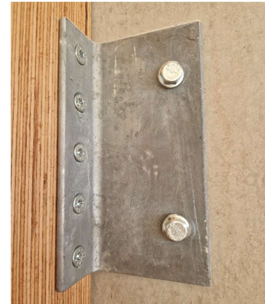
Finished job site
