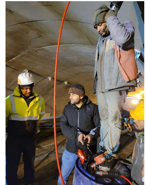
Baseplate application and Hilti anchors at jobsite
