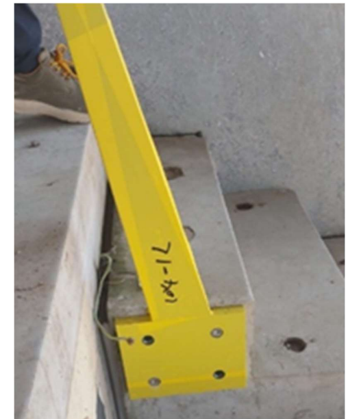
Ongoing anchor installation and finished baseplate connection
