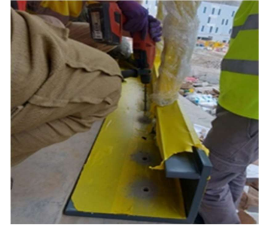
Ongoing anchor installation and finished baseplate connection
