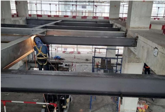
Application Details: Baseplate-beam-column joint
