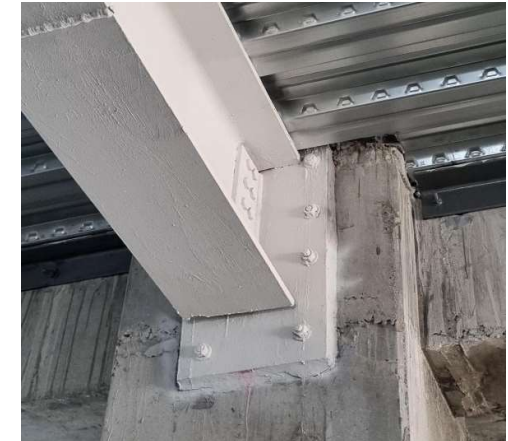
Finished baseplate connection and demonstration at site
