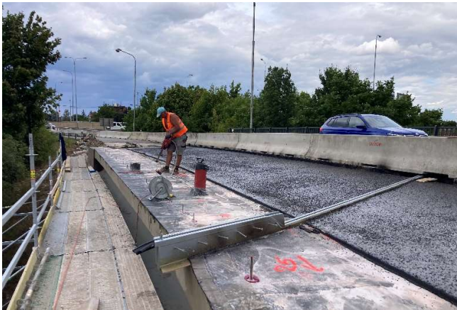
Application Details: Waterproofing connection
