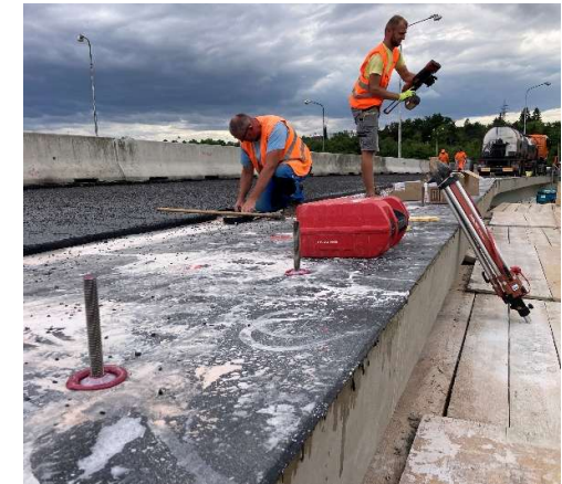
Ongoing anchor installation and finished post-installed connection
