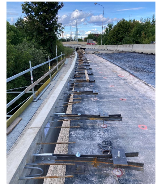
Ongoing anchor installation and finished post-installed connection
